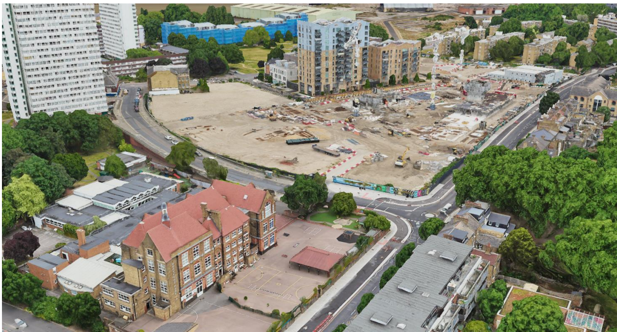
Looking eastwards towards Oxestalls Road
