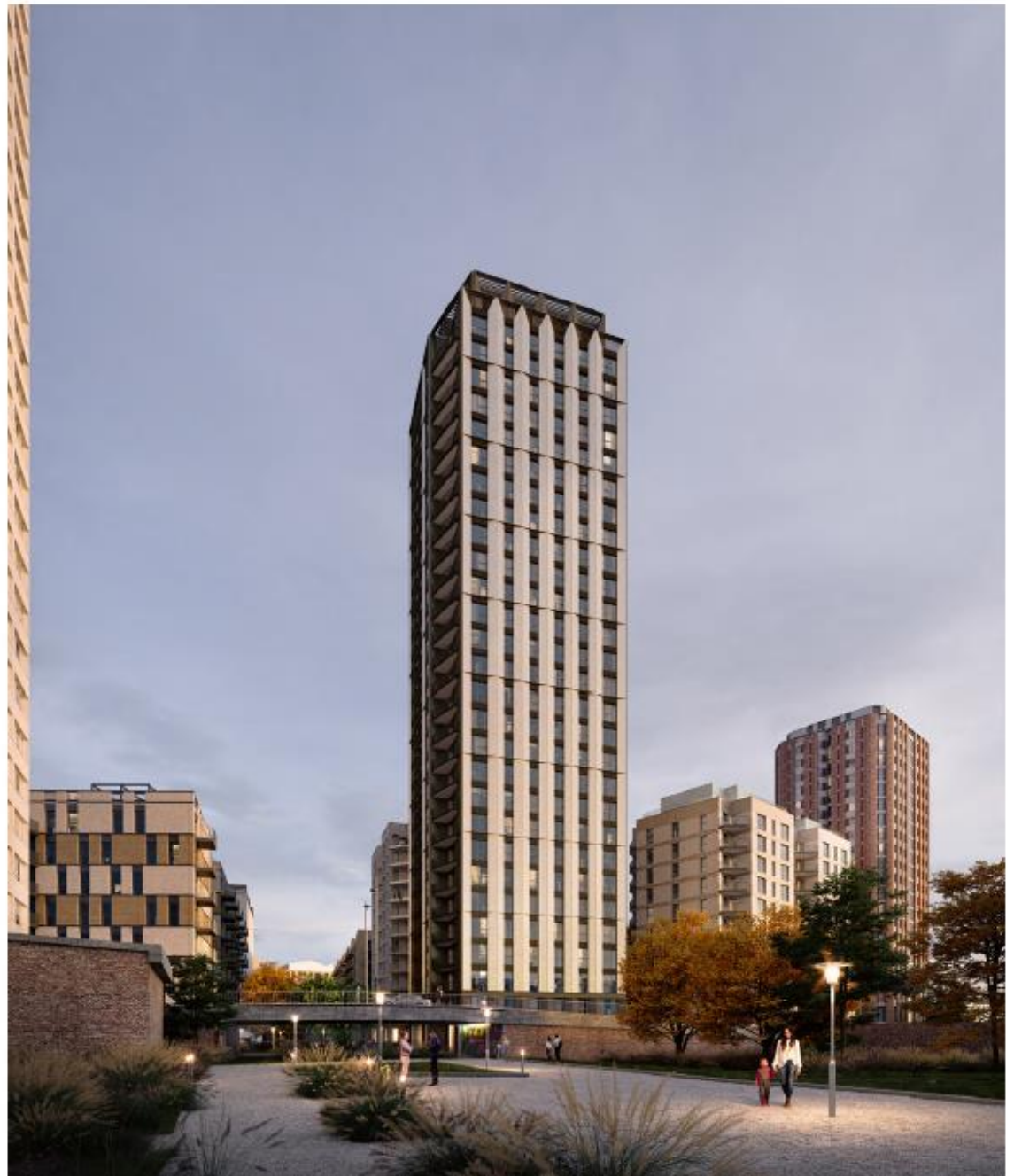
Waterline Tower (5C)
